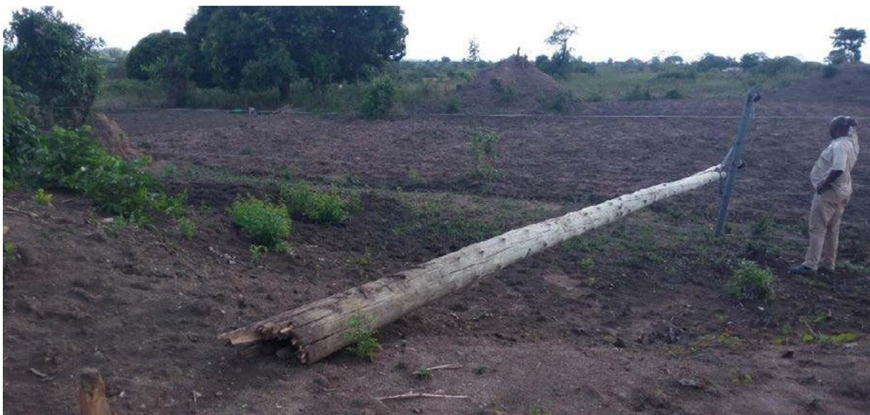
Figure 5. Collapsed electricity pole on farmland along the Kampala–Tirinyi highway that crosses Pallisa district
